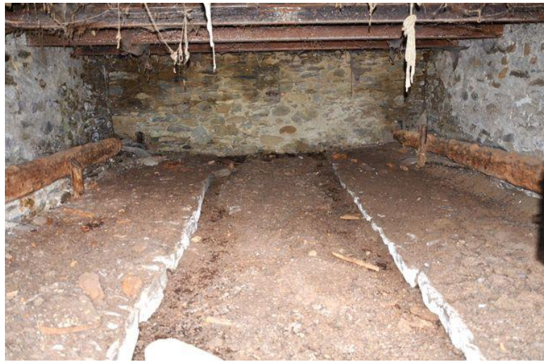
Innenraum Erdgeschoss / interno piano terra
