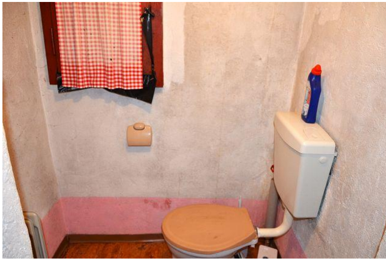
Bad – WC / bagno – WC
