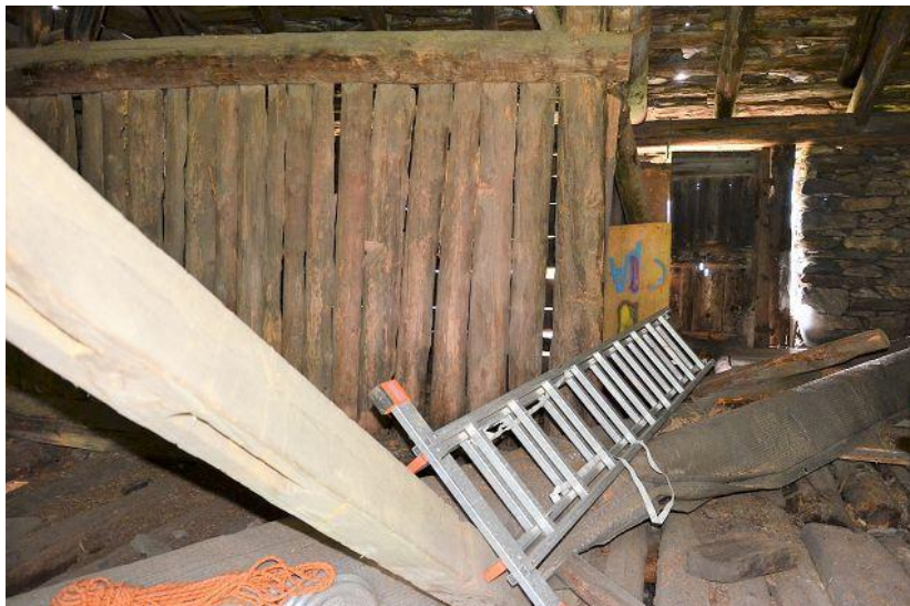
Scheuneninnenräume / interni stalla
