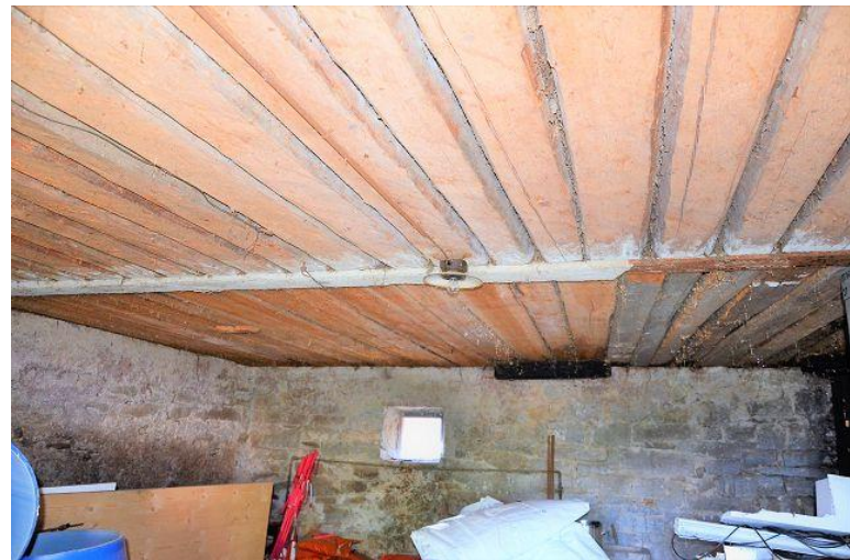
Innenraum Erdgeschoss / interno piano terra
