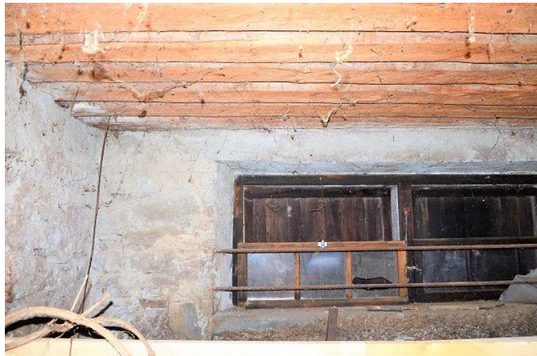
Innenraum Erdgeschoss / interno piano terra
