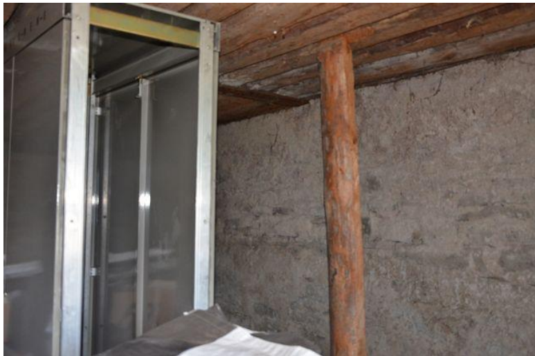
Innenraum Erdgeschoss / interno piano terra
