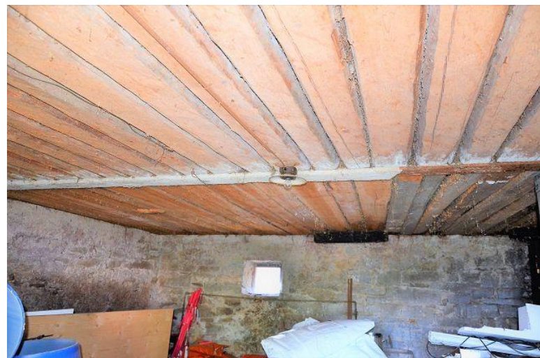
Innenraum Erdgeschoss / interno piano terra
